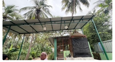
The covered ritual pavilion and shrine
